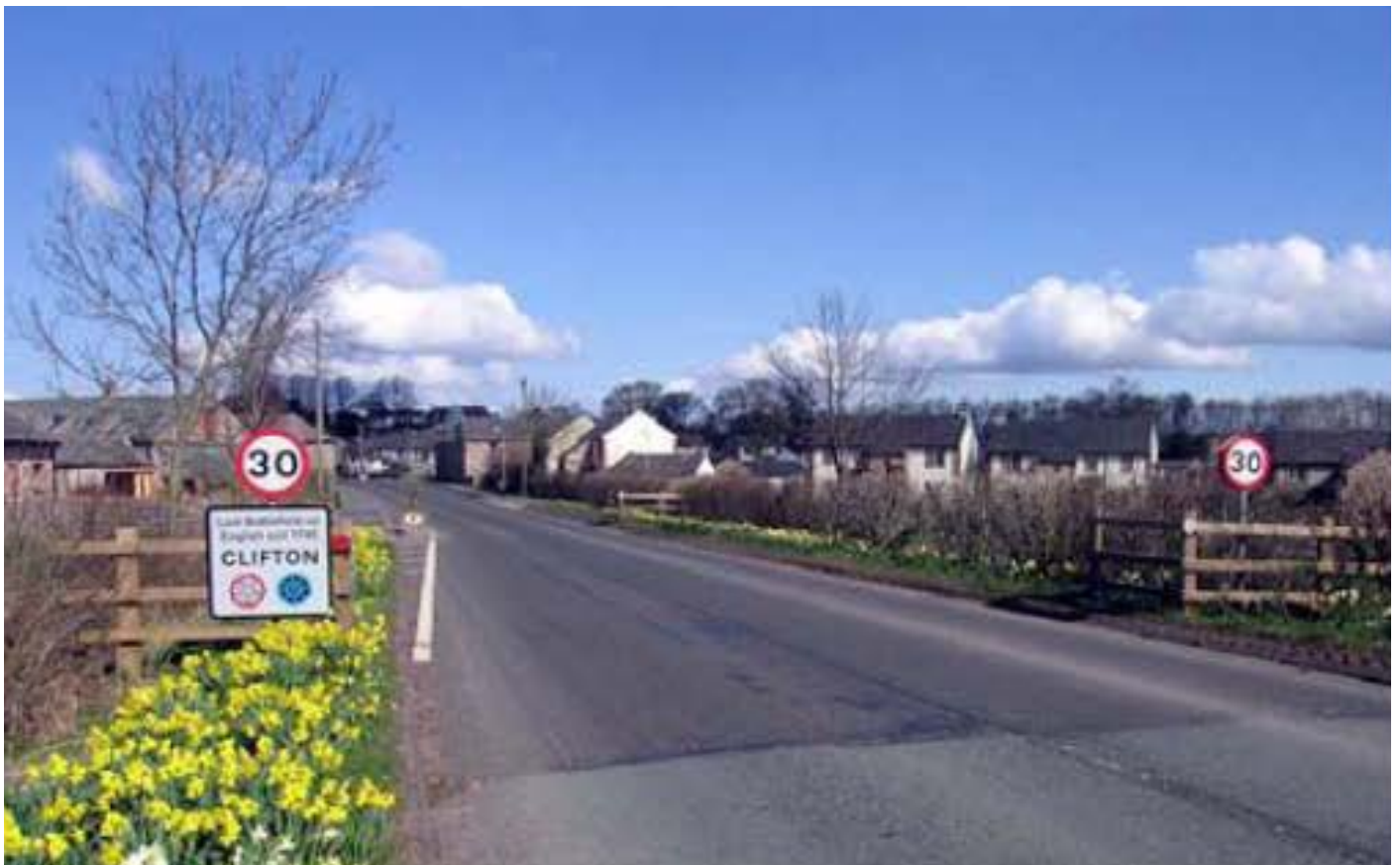
FIGURE 16_A EXAMPLE THROUGH THE A6 THROUGH CLIFTON VILLAGE IN CUMBRIA - A 'GARDEN GATE' ON THE MAIN APPROACH TO THE VILLAGE PSYCHOLOGICALLY SLOWS DOWN DRIVERS
